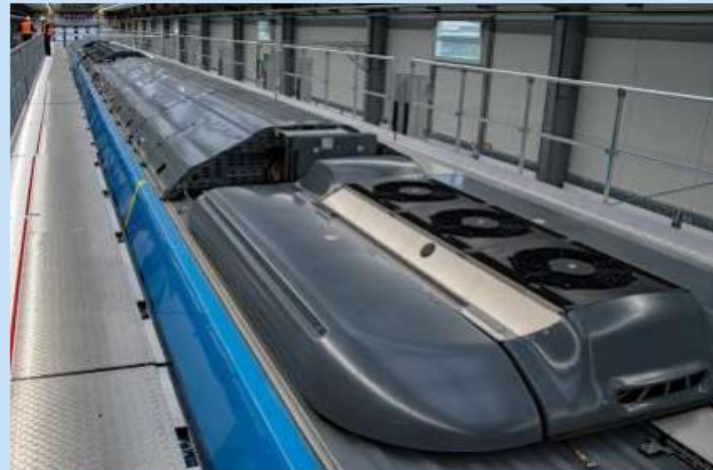
HVAC and Hydrogen tanks
